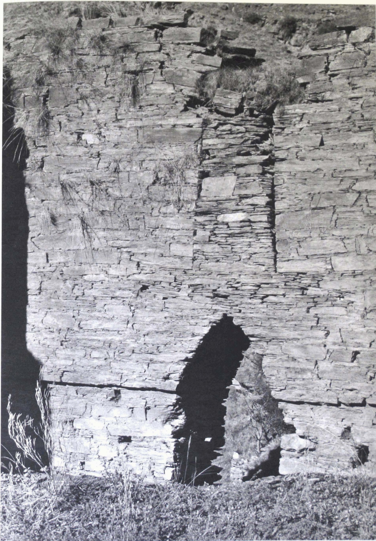
Temple Site, Assembly Hall, North Wall
